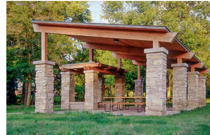
Two roof styles could be considered to optimize the potential number of solar panels. Photos from Vermont Timber Works.
