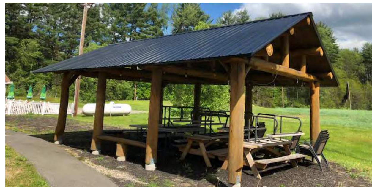
Timber frame pavilion with gravel instead of a concrete pad for a base may be less expensive. Photo from Richard Gallow.
