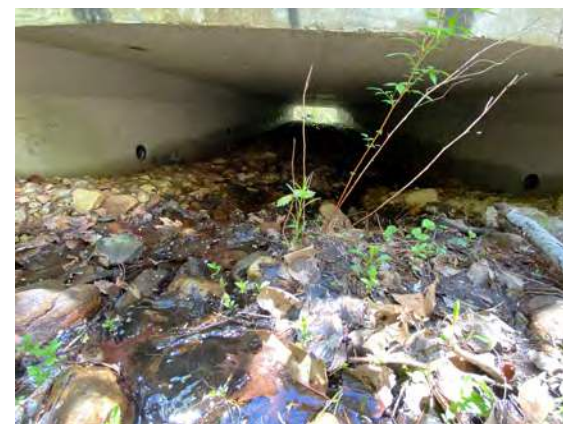
Culvert under Watkins Way
