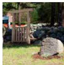
A new gate and a stone monument were part of the Fitchburg Town Pound restoration project.
