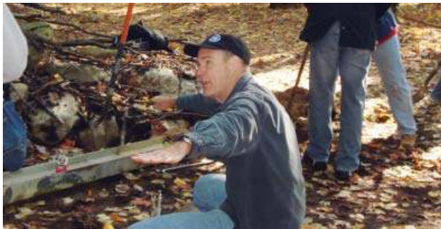
NCLT Director, Jim Walsh led a group of volunteers from DRS Power Technology in a trail work day which included the installation of bollards and chains to prevent unauthorized access to Crocker CA trails by motor vehicles.
