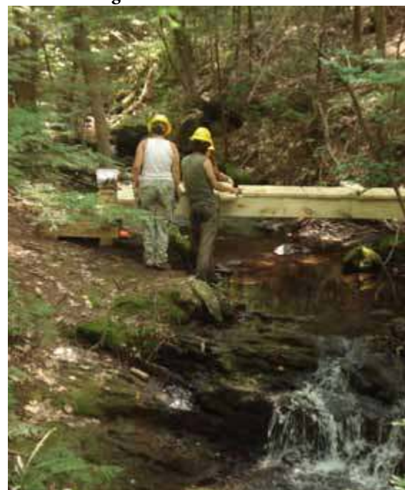
SCA bridge construction on Falulah Brook
